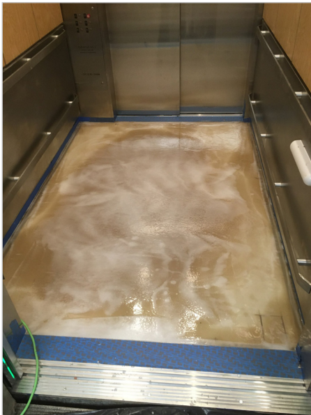
Left: Primer and 30 mesh sand have been applied over cleanly sanded plywood.
