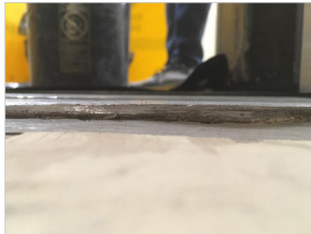
Left: Primer and 30 mesh sand have been applied over cleanly sanded plywood.
