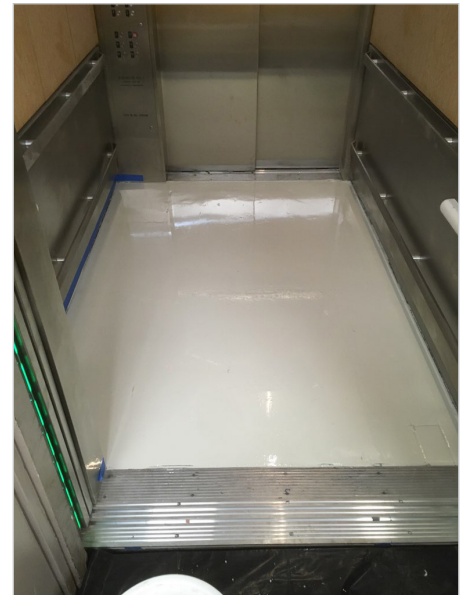
Above: Joint where plywood meets the edge of the cab has been sealed.
